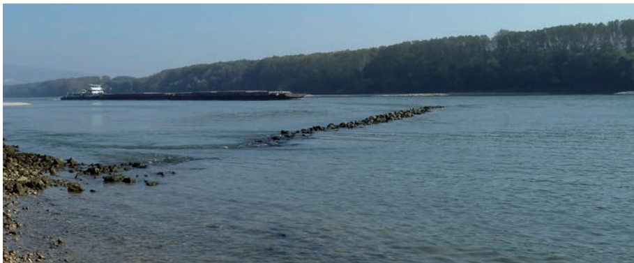
Declining groyne, i.e. adjusted to the river's flow direction, for river regulation at low water levels
