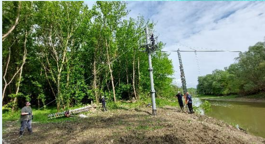
Installation of equipment to measure water levels, discharges and suspended sediment
