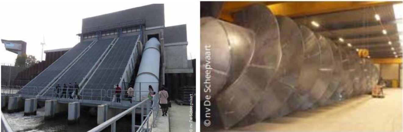
Figure 50: Overview of the four Archimedes screws installed in one of the six lock systems. The last screw on the right is equipped with a casing to avoid harming fish (left). An Archimedes screw in production (right).
