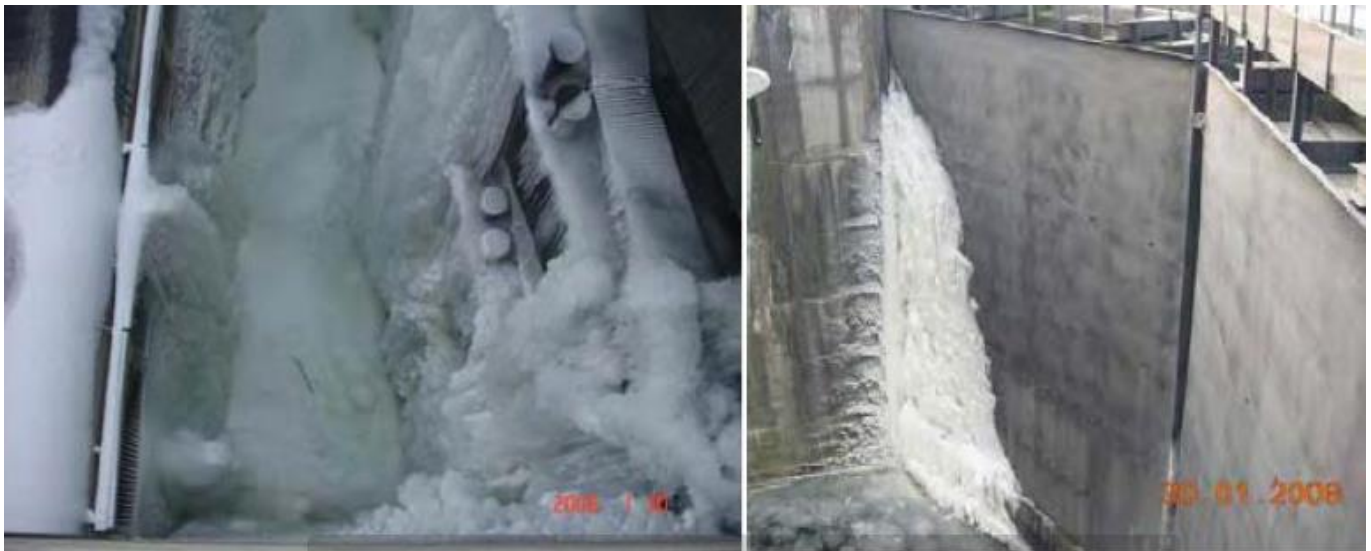
Figure 21: Ice occurrence in locks on the Danube preventing their operation. The figure left was taken in the year 2006. The figure right was taken in the year 2008. Source: viadonau.
