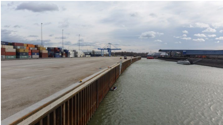
Land reclamation and reduction of the port basin through embankment at port Freudenau (2012-2015)
