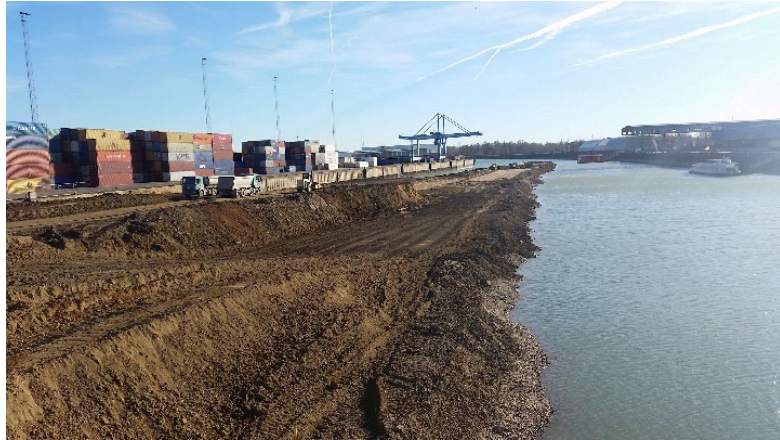
Land reclamation and reduction of the port basin through embankment at port Freudenau (2012-2015)
