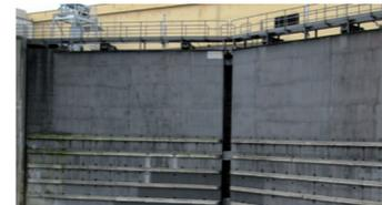
**Mitre gate** double-leaf gate at the downstream end of the lock
