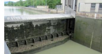
**Downstream lock head** Gate construction at the downstream end of the lock
