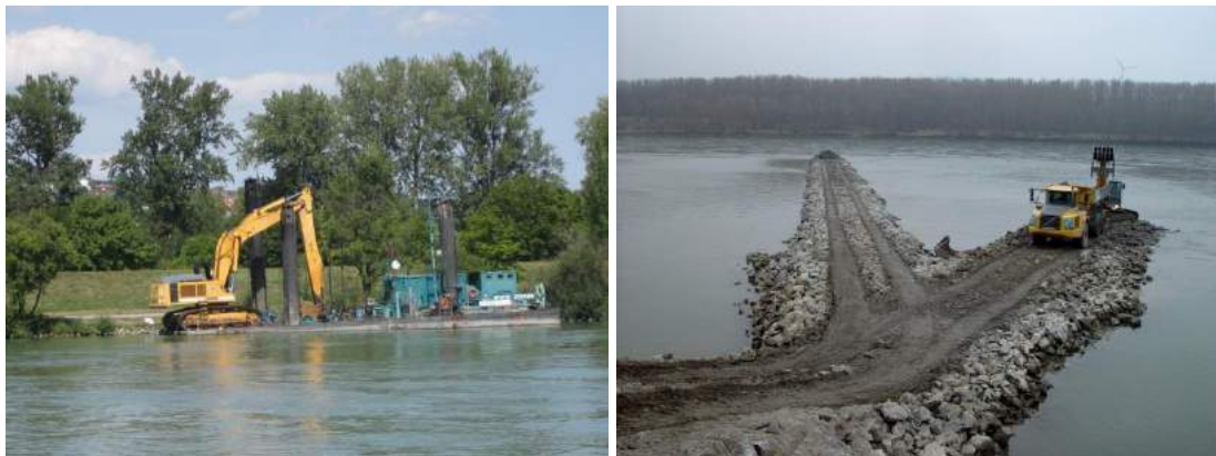
Figure 2: Maintenance works and groyne adaption on the Austrian stretch of the Danube (free-flowing sections Wachau and east of Vienna)
